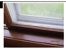
**LOCATION:** Bedroom, Back Left **SYSTEM:** Interior **CONDITION:** Window unit has damaged weatherstripping
