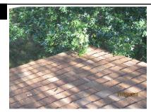
**LOCATION:** Exterior Right Side **SYSTEM:** Exterior **CONDITION:** Tree branches are too near to the roof surface
